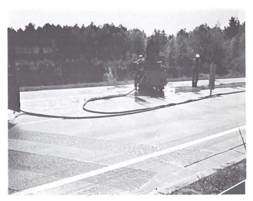
(Longitudina Igrooves will also increase friction between Tyre and Toad surface. They are theaper to make than transverse grooves. Yet this solution is not recommended because of the adverse effects on motor cyclists 'riding behaviour')
