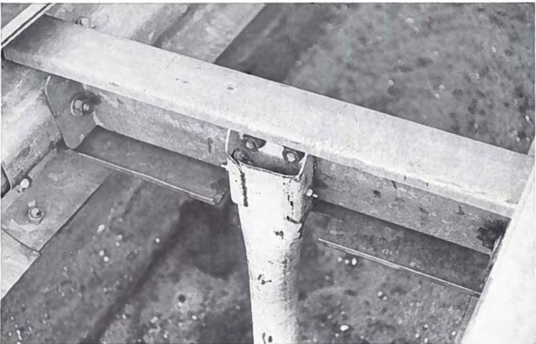
Figure 23. Rupture device in post-to-spacer fixture.
