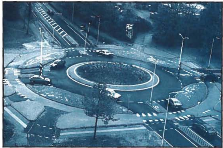
Roundabout with separate cycle track in the Dutch town Enschede: The bicyclists have right of way.
