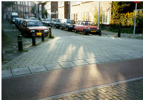
Figure 6.1. Raised pedestrian crossing in Utrecht, the Netherlands.
