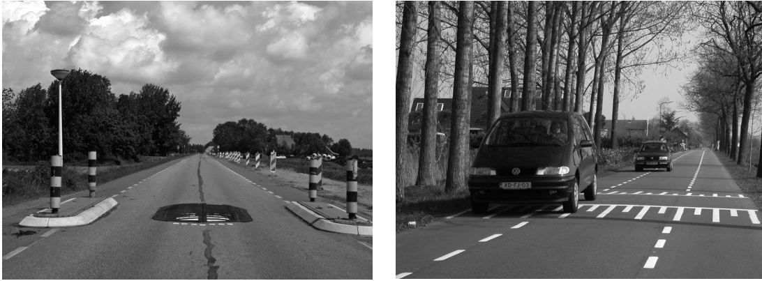
Figures 8.4. Example of driver friendly (left) and not driver friendly (right) speed measure according to CROW-publications (CROW, 2002c; 2002d; 2007b; Goudappel-Coffeng, 1999) (Photography: Robert Louwerse).
