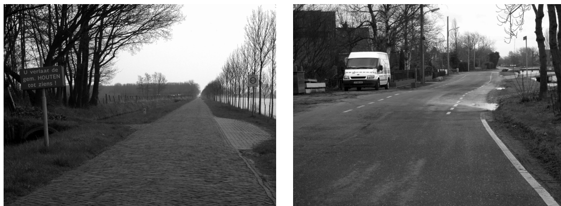
Figure 8.3. Example of consistent (left) and not consistent (right) road transition (Photography: Robert Louwerse).
