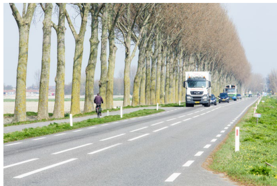
Figure 3. Rural distributor road, without physical separation of driving directions, with double centre lines (Photo: Paul Voorham).
